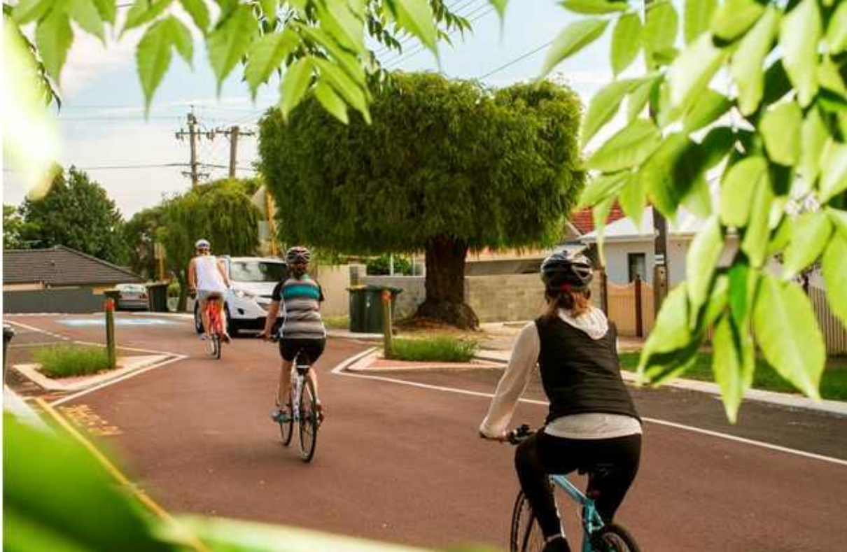
Figure 3.2 – Cycle Street – Example from Perth where red asphalt is used to highlight the cycle street (Source: Department of Transport Western Australia)
