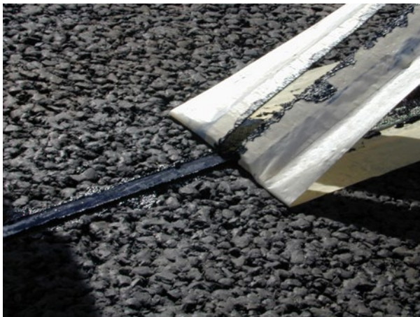
Figure 7.4.4.2(g) – Piezoelectric installation details (removal of sealant excess)
