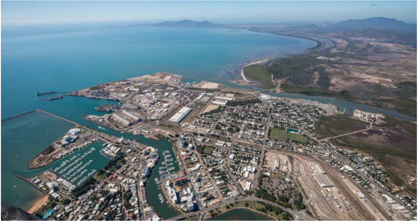
Aerial of the Port of Townsville and the Townsville State Development Area
