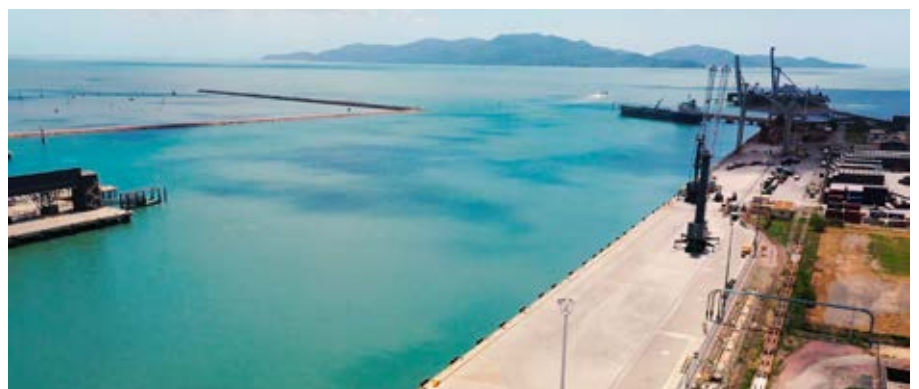
Newly upgraded Berth 4 quay-line
