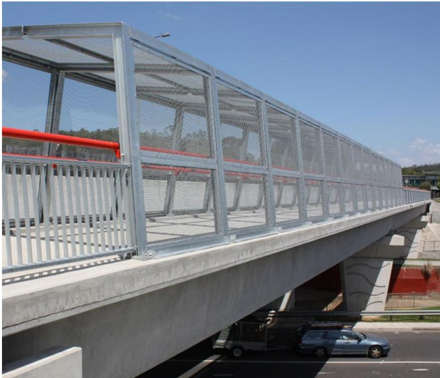
Note the provision of angle cover strip to close gap at base of screens.
