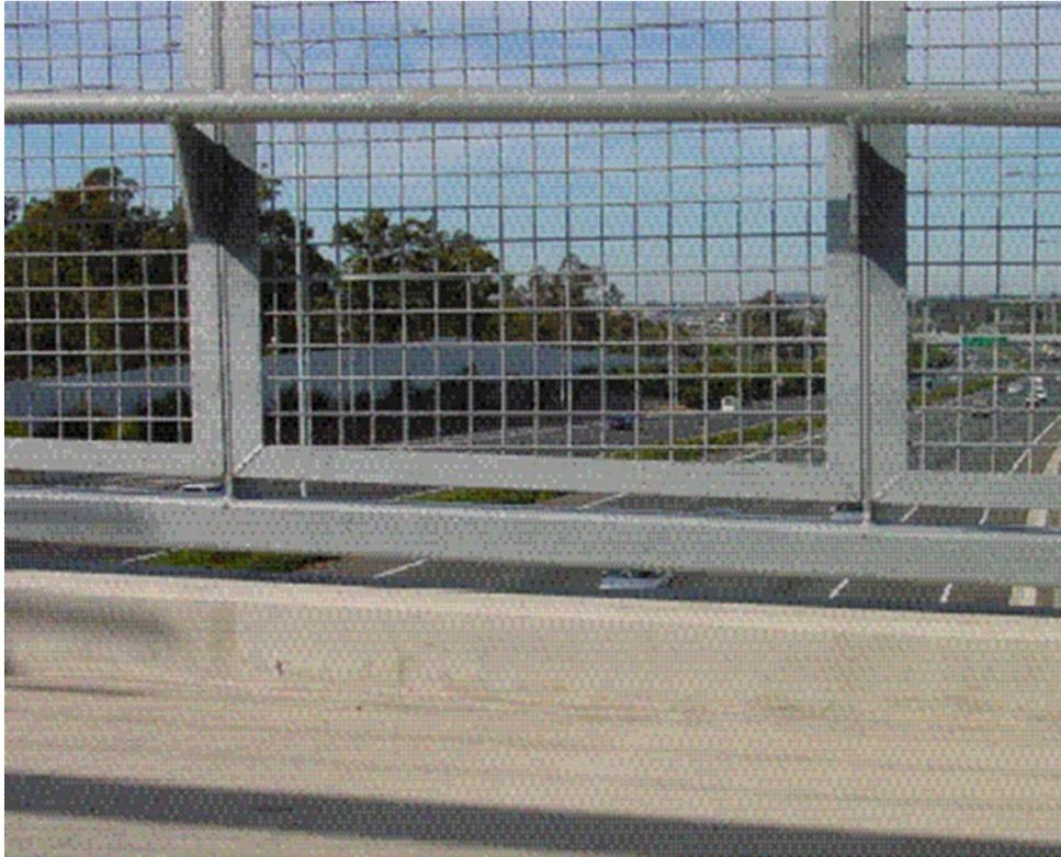
Note the 50 mm high opening along bottom edge of screen – this should be avoided.
