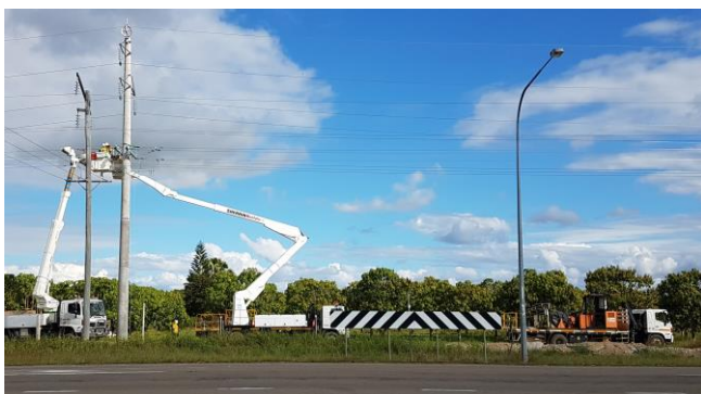
Stringing HV lines – southern end of project
