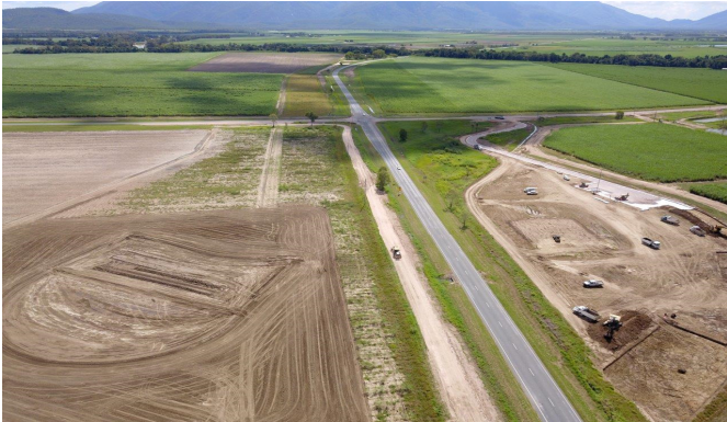
Clearing of Hodel Road overpass area (looking towards Townsville)
