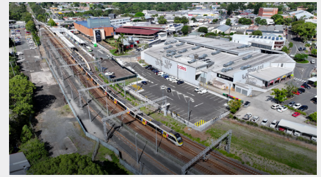
Image: Upgraded Nambour station park 'n' ride (TMR)
