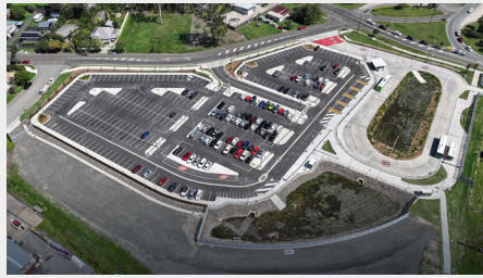
Image: Upgraded Landsborough station park 'n' ride (TMR)
