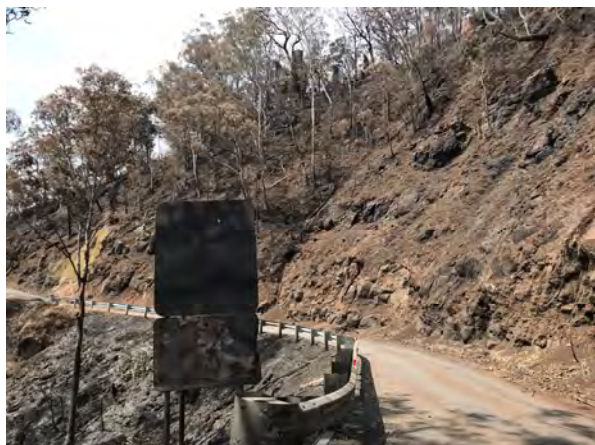
Above: Following the fire in September 2019.
