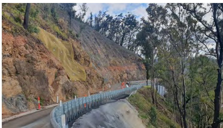
Above: Drape mesh, rock-fall protection and guardrail installed, June 2020
