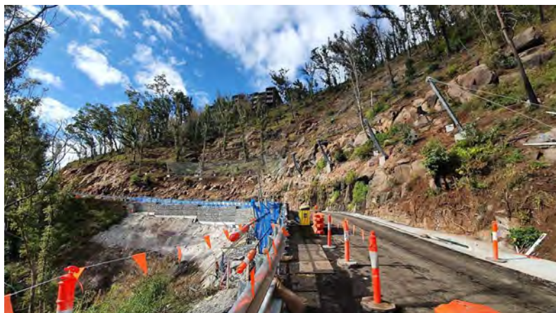
Above: Progress in June 2020.
