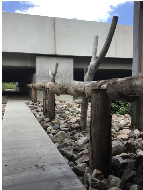
Figure 9 and 10. Fauna structures installed at Mooloolah River
