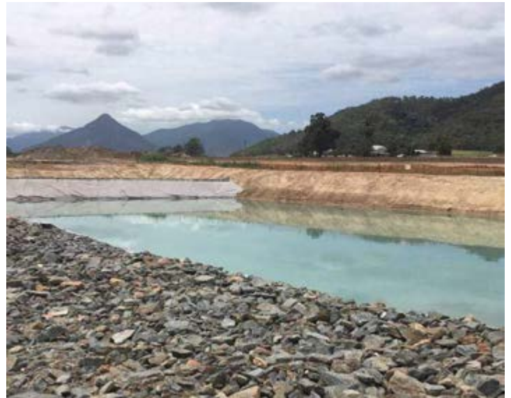
Sediment pond at Wrights Creek (North).
