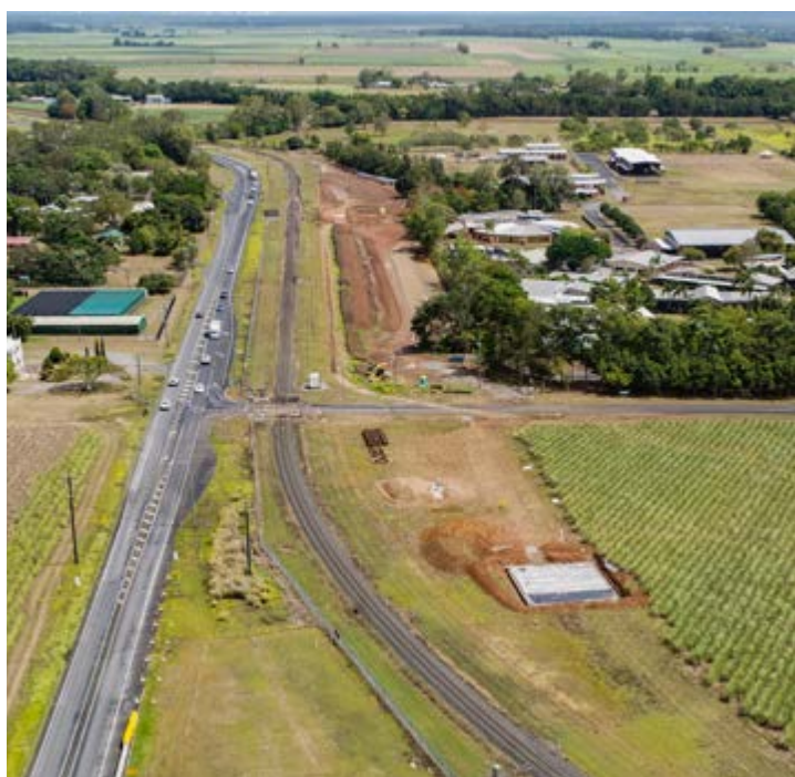
Realignment of Queensland Rail North Coast Line at Maher Road.
