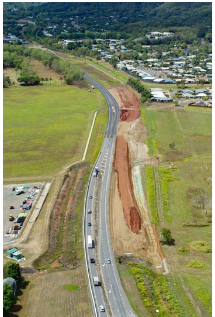
Construction of Bruce Highway duplication and cycleway at Draper Road South.
