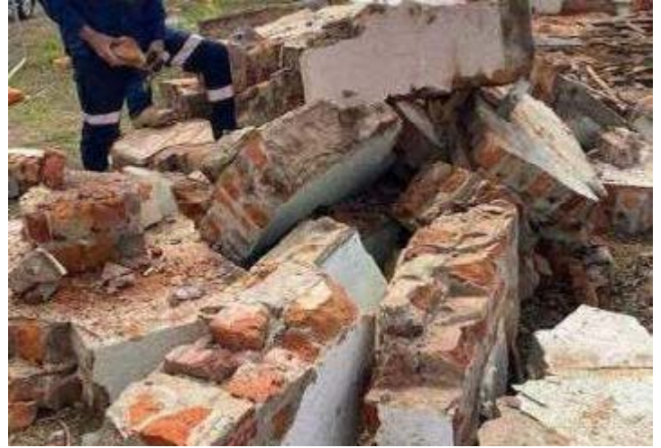
Bricks recovered from demolished farmhouse.
