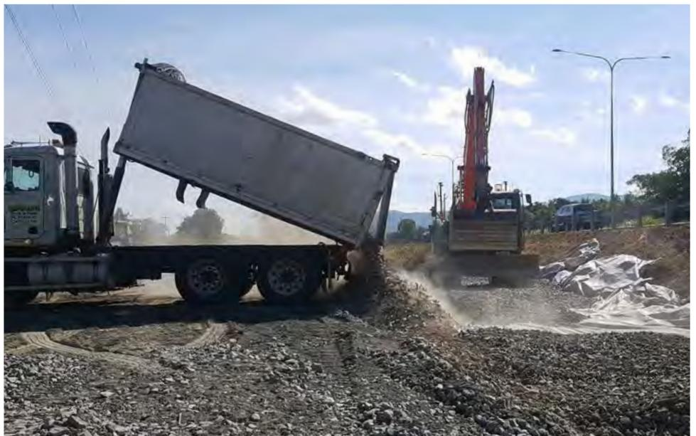
*Installation of the rock drainage layer adjacent to the Bruce Highway at Chinaman Creek.*
