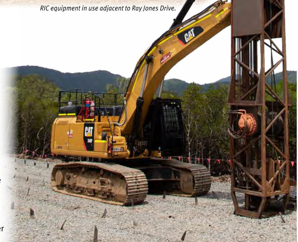
*The wick drain installation machine installs drains 1.5m to 2m apart.*
