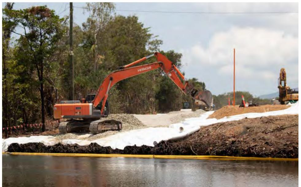
Excavator spreading rock fill over geofabric next to Chinaman Creek.
