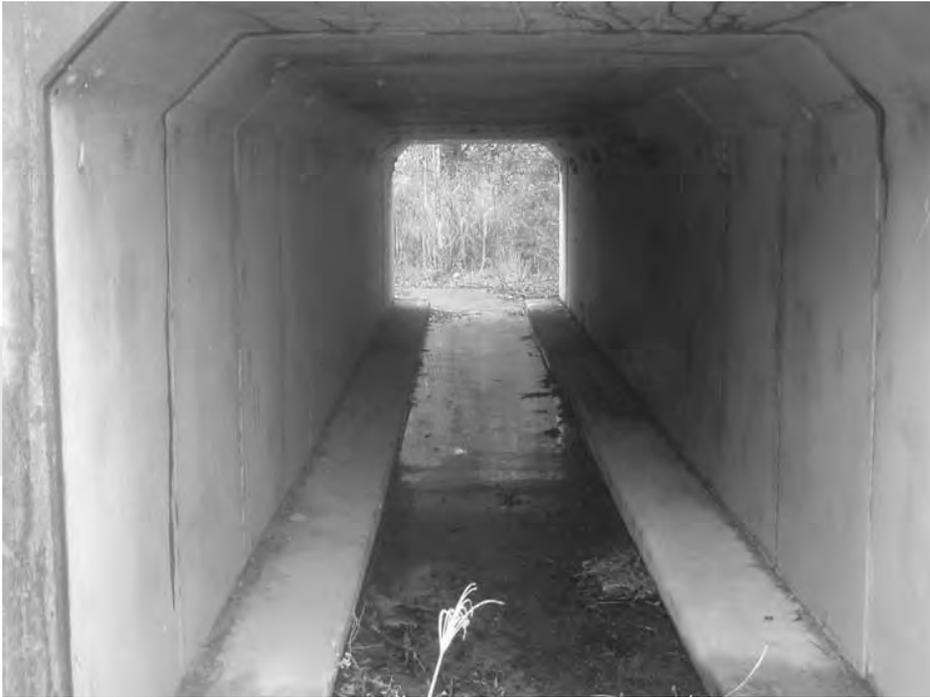
**Plate 1. Culvert with dry ledges**
