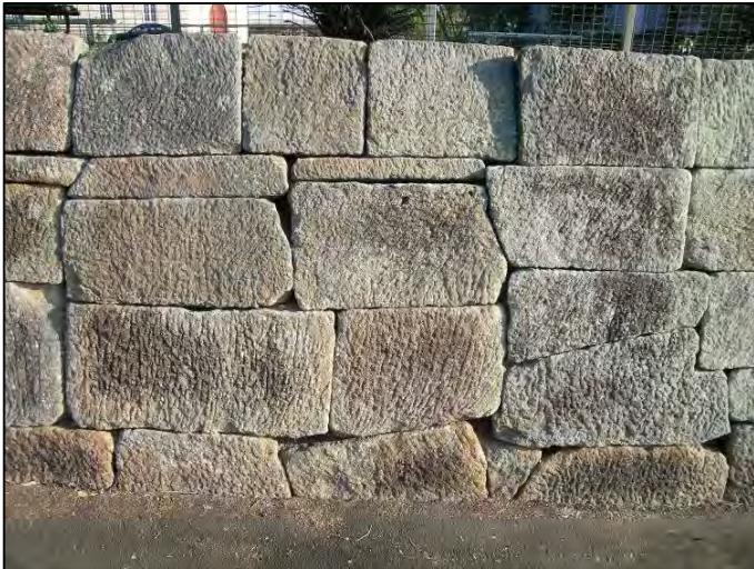
Figure 12. Boundary wall at Surface Hill Uniting Church, Gympie.
