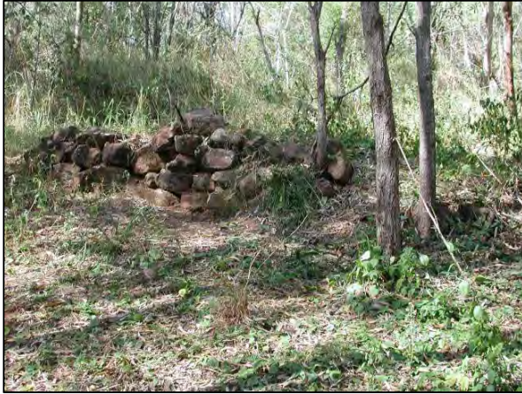
Figure 4 - Western face of Feature F2 shows the dry-stone wall of the structure
