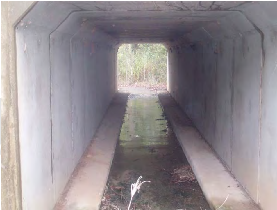
Plate 1. Culvert with dry ledges
