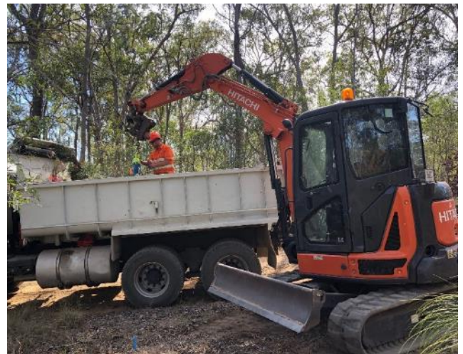
Plate 17. Shows bogie tipper and 5t excavator from Ace of Spades.
