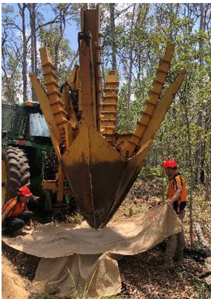
Plate 22. Shows the spade with root ball and plant inside lowering plant into cage lined with hessian.
