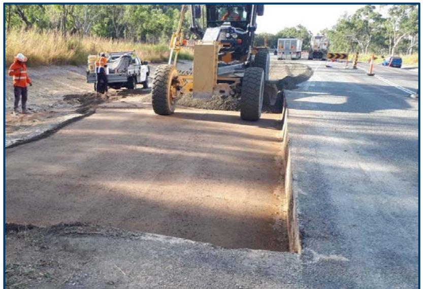
Existing sections of pavement have been excavated in preparation for being widened and reconstructed.
