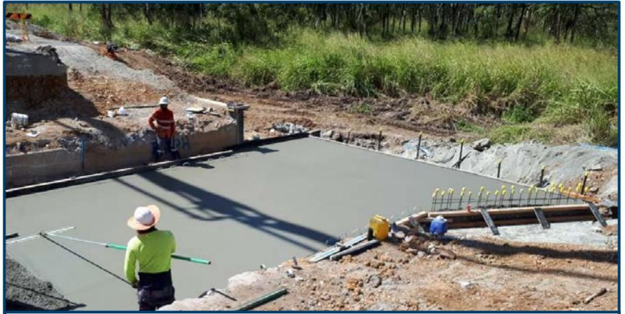
Culvert banks are continuing to be constructed throughout the project, ahead of pavement widening.
