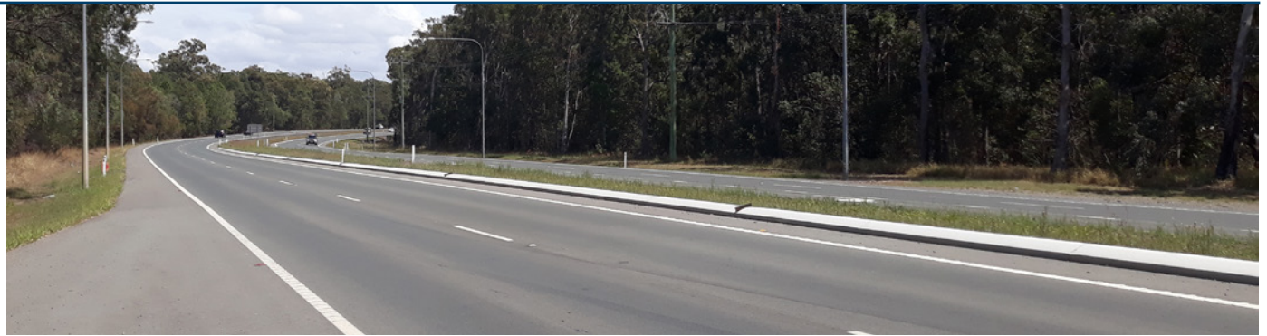
An existing 4-lane median divided section of Bribie Island Road
