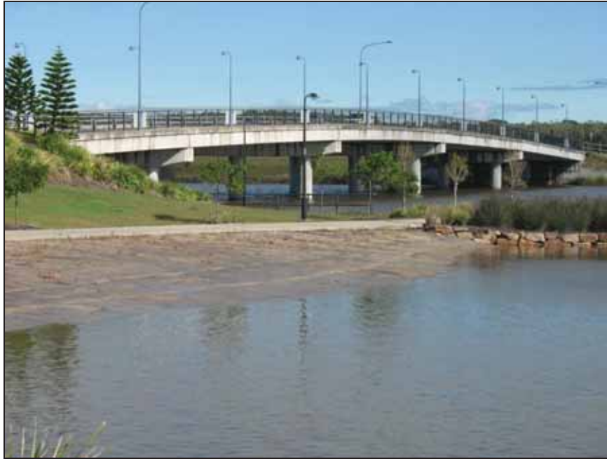
Photo 5-4: Lake Kawana Bridge (East)
