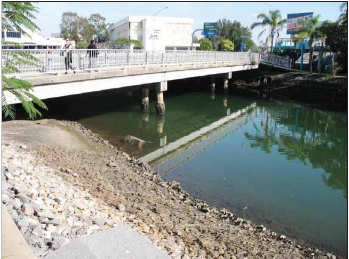
Photo 5-8: Cornmeal Creek Bridge
