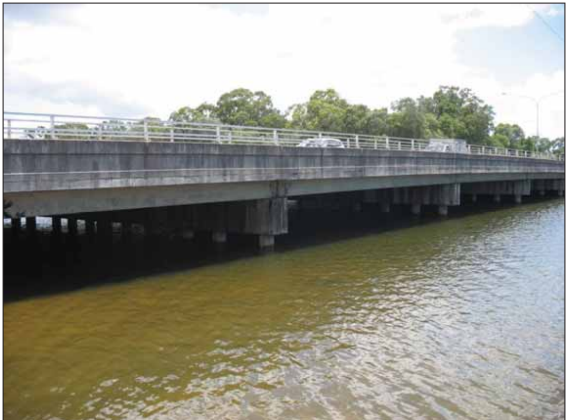
Photo 5-2: Currimundi Creek Bridge
