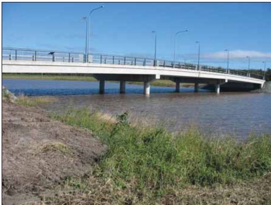
Photo 5-5: Lake Kawana Bridge (West)
