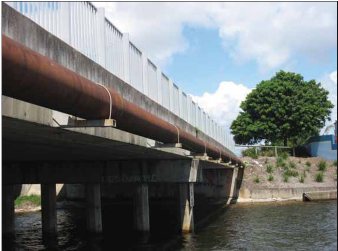
Photo 5-3: Tokara Canal Bridge
