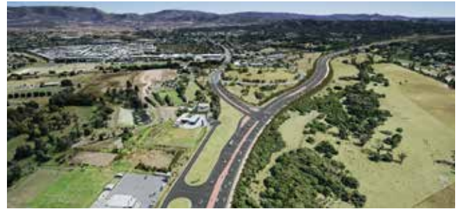
Nerang-Broadbeach Road intersection
