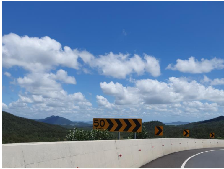
Figure 6: Reinforced earth embankment vegetation growing behind barrier
