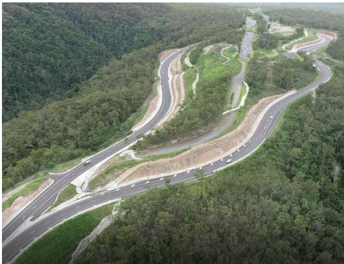
Figure 3: Split carriageway (looking uphill)
