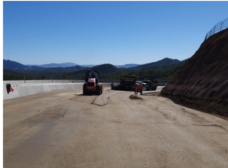
Figure 12: Cemented treated base construction
