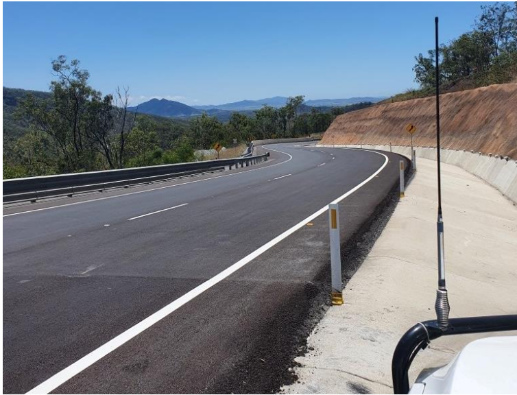
Figure 9: MC001 open to traffic
