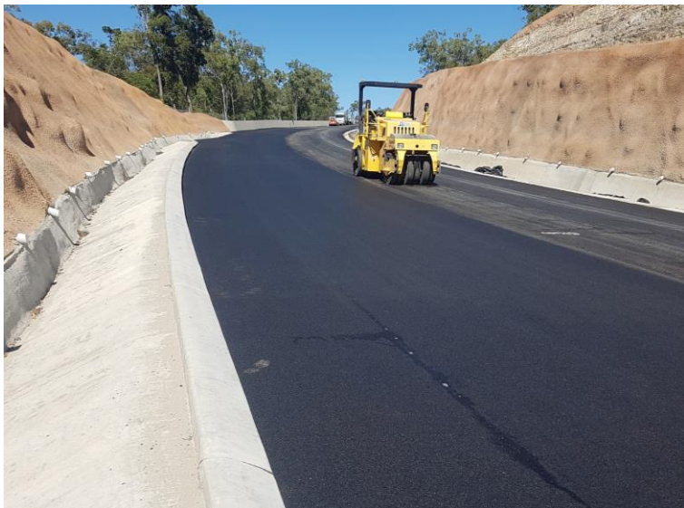
Figure 11: MC002 Asphalt placement
