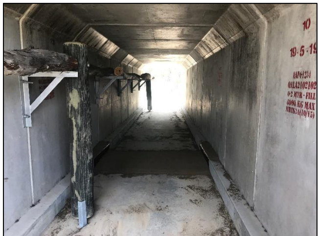
Plate 4: Sand Plot 2 set up in Culvert 1.
