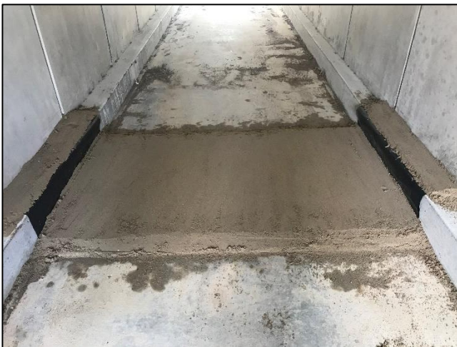
Plate 1: Sand Plot 6 set up in Culvert 3.
