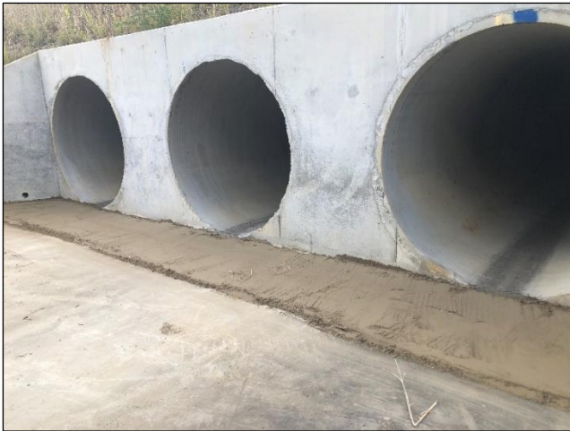
Plate 3: Culvert Sand Plot
