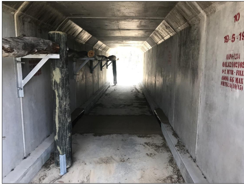
Photo 36: Fauna Furniture in Box Culvert
