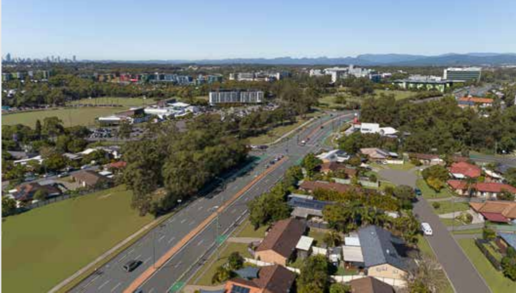
Artist's Impression: Olsen Avenue southbound to Gold Coast Hospital and Griffith University.
