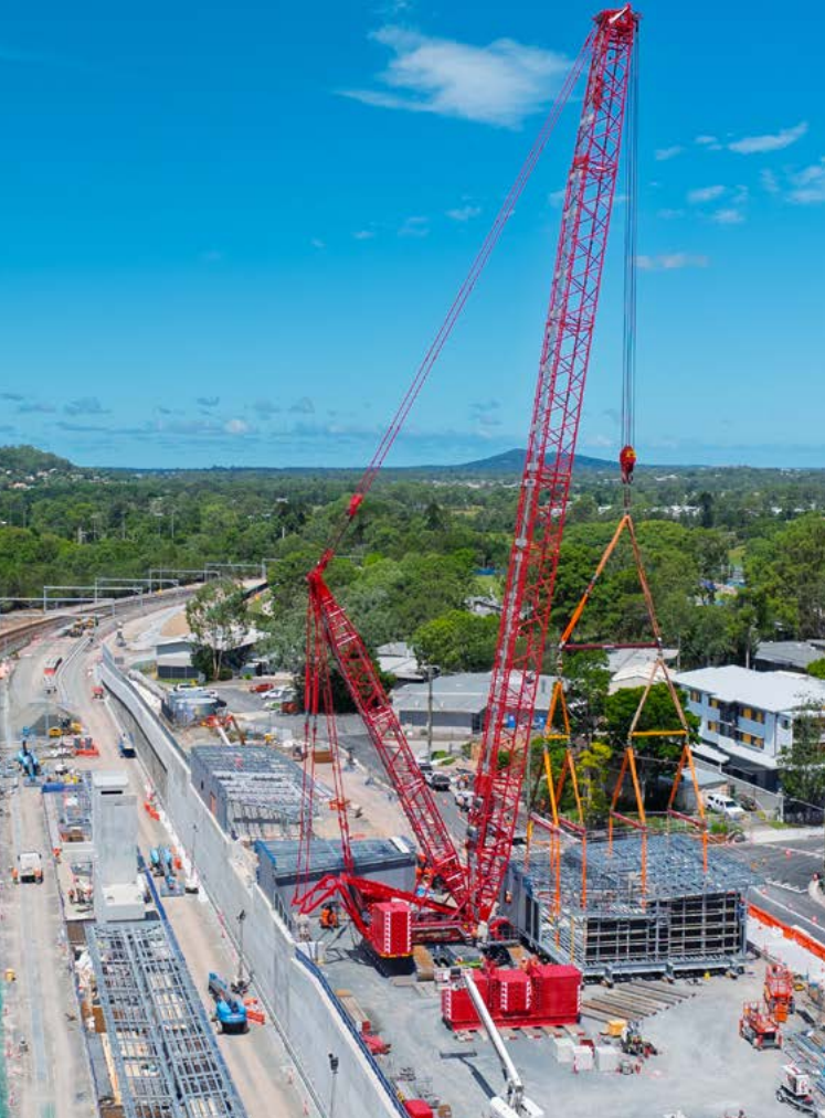
A 480-tonne crane was used to lift the first section of the new Loganlea pedestrian footbridge into place
