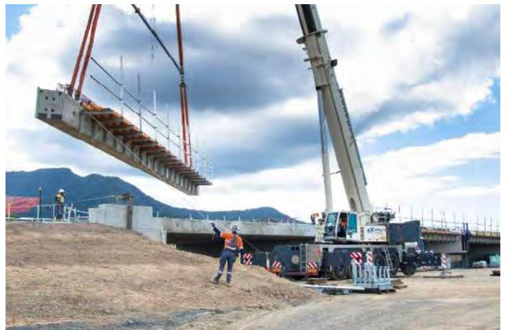
*Installation of bridge deck units at Avondale Creek bridge.*
