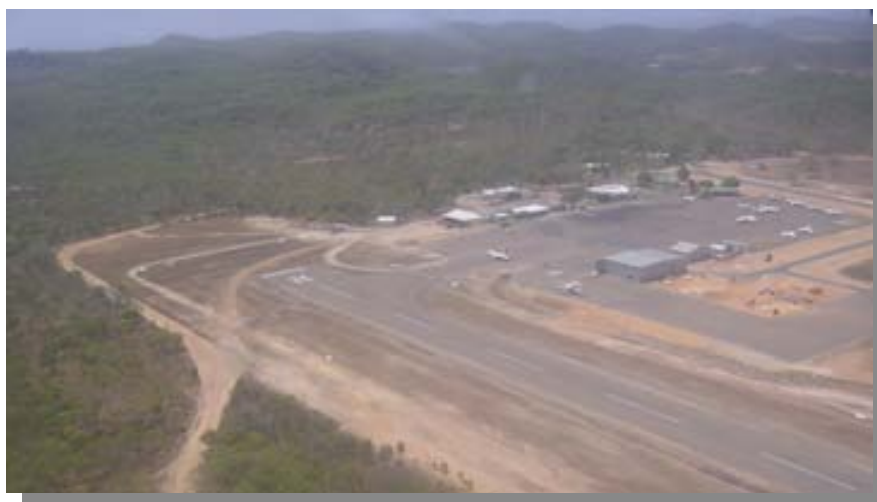
Figure 3.14 Horn Island Airport
