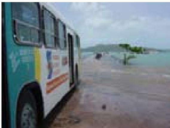
Figure 4.7 King Tide at Horn Island Ferry Jetty
