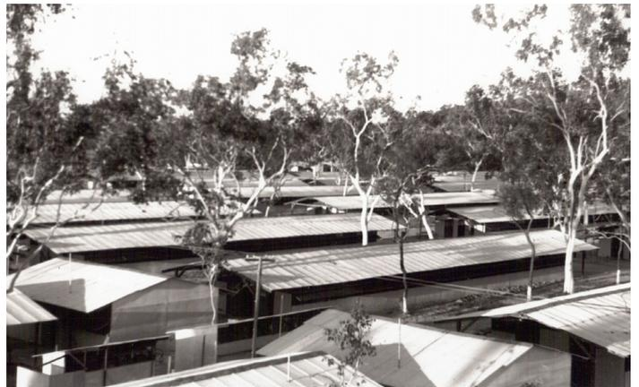
*Prefabricated tents were insulated and included adjustable shutters, a wooden floor and a corrugated iron roof.*
