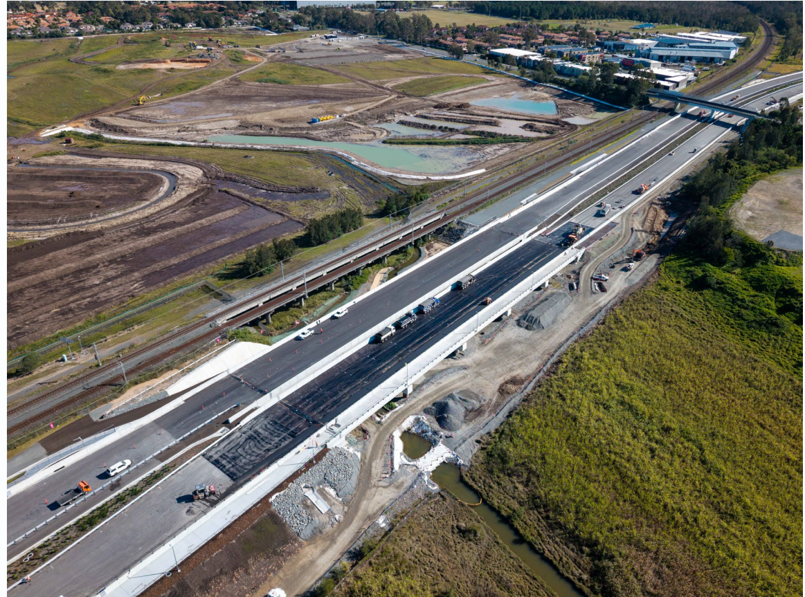
New Coomera River bridge delivered as part of Coomera Connector Stage 1
