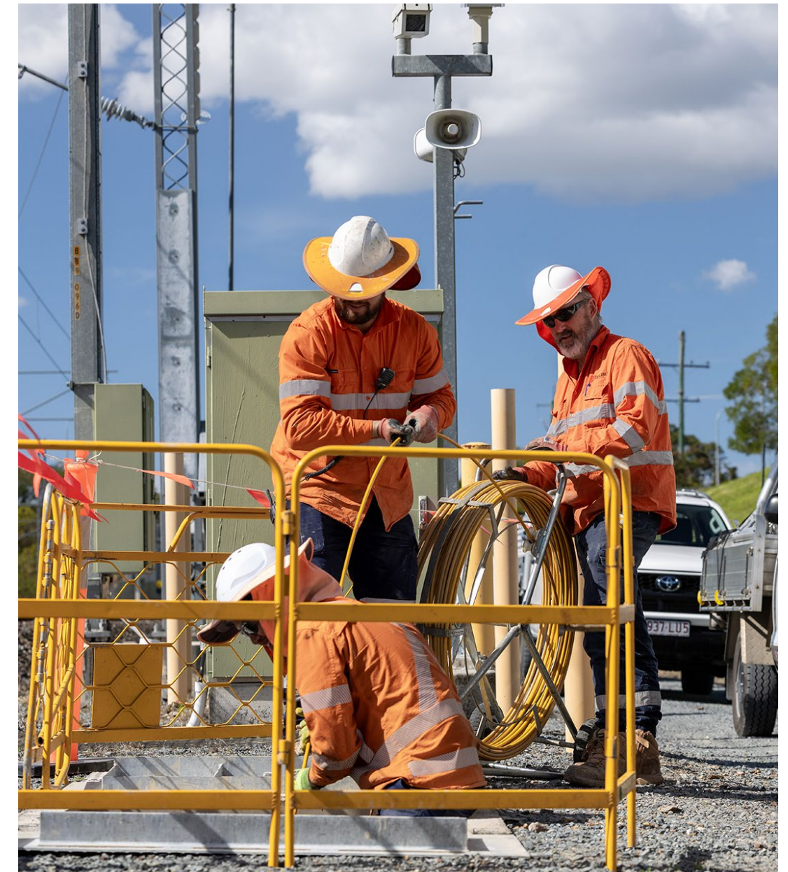
Installing new fibre optic cable for ETCS on the Beenleigh to Varsity Lakes project.
