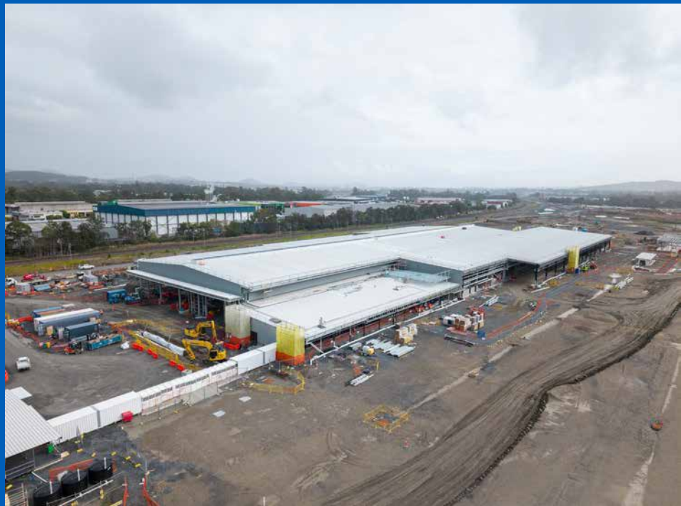
Ormeau rail facility - May 2026
