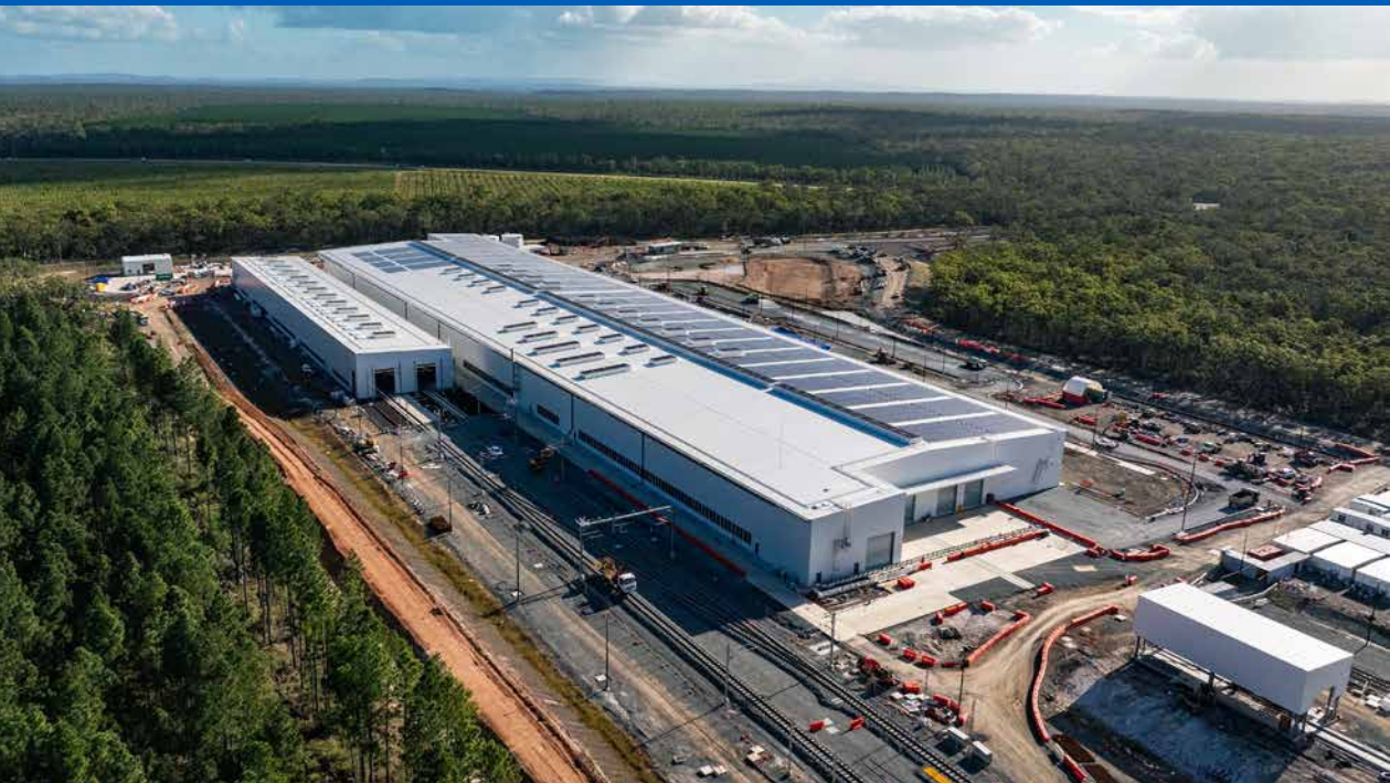
Torbanlea train manufacturing facility - May 2026
