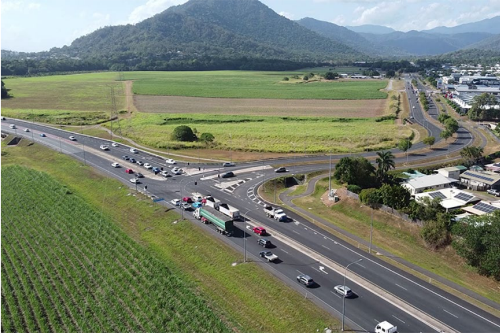
The Cairns Western Arterial Road, Redlynch Connector Road
