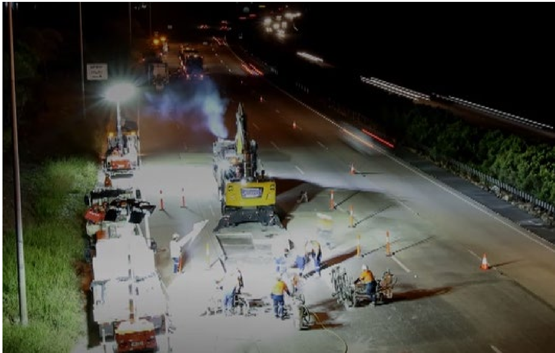
Pacific Motorway, M1 concrete slab replacement night works
