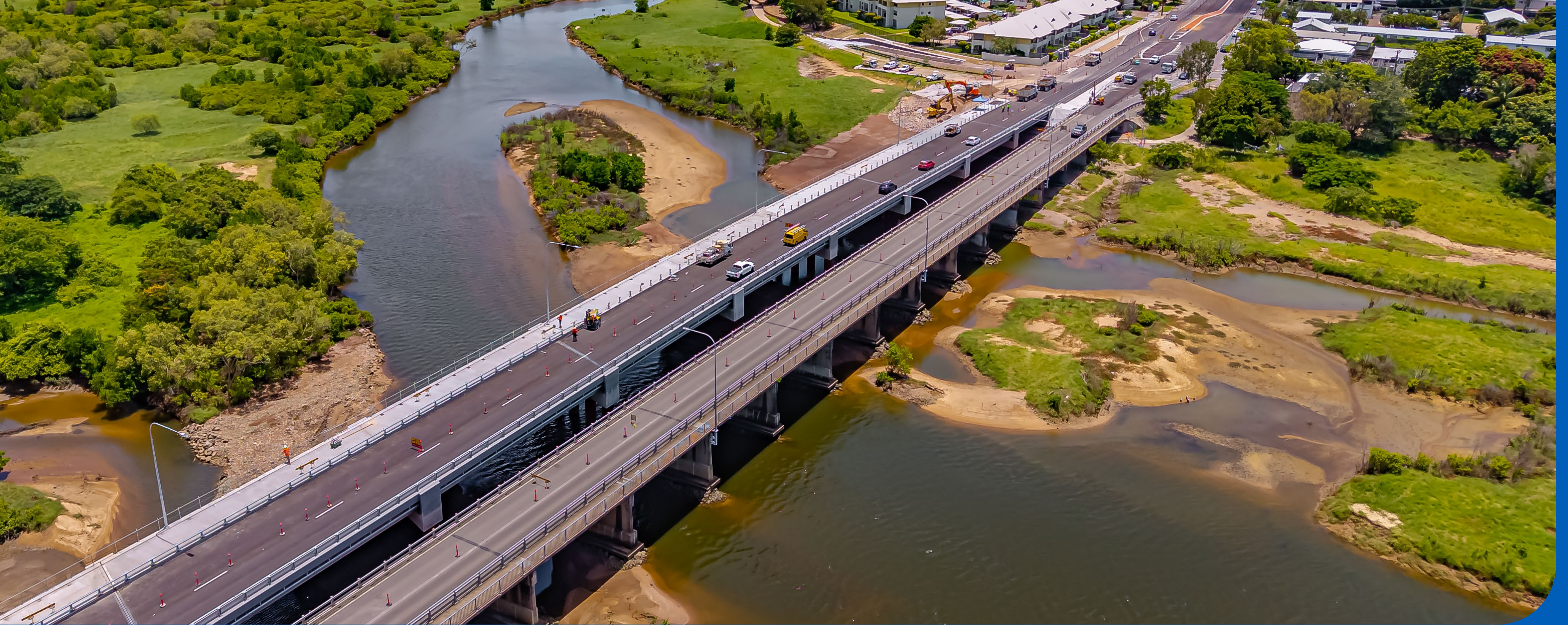
Nearly complete upgrade to Bowen Road Bridge on Townsville Connection Road (Stuart Drive) in Idalia.
