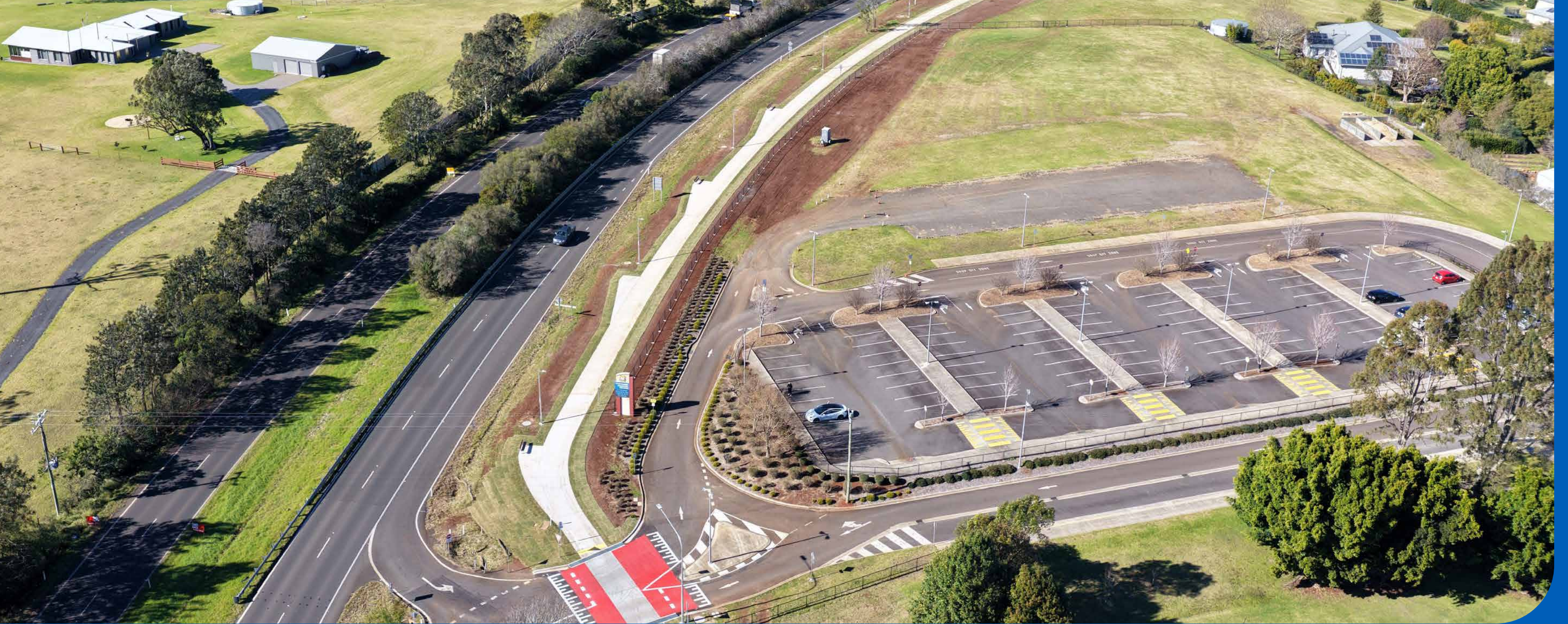
New priority pedestrian crossing at the entrance to Toowoomba Christian College, part of the New England Highway Bikeway, Highfields to Toowoomba CBD Stage 2.
