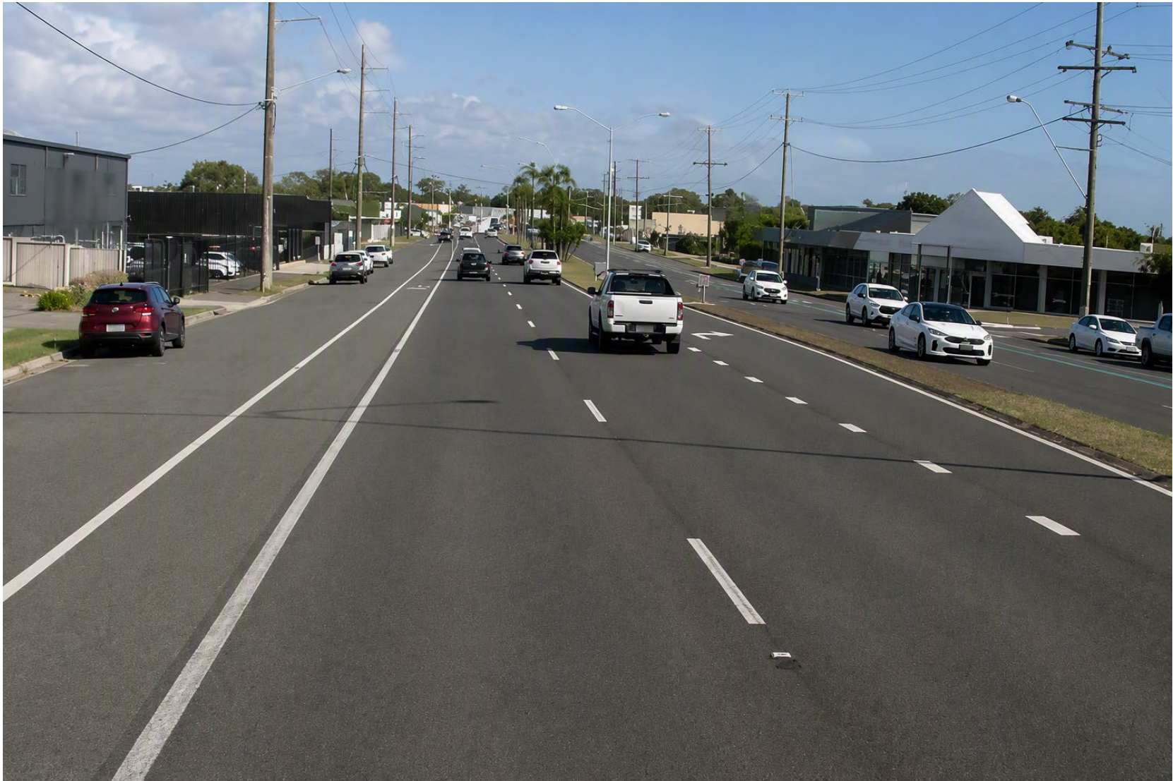
Nicklin Way, Coora Crescent intersection (Currimundi)
