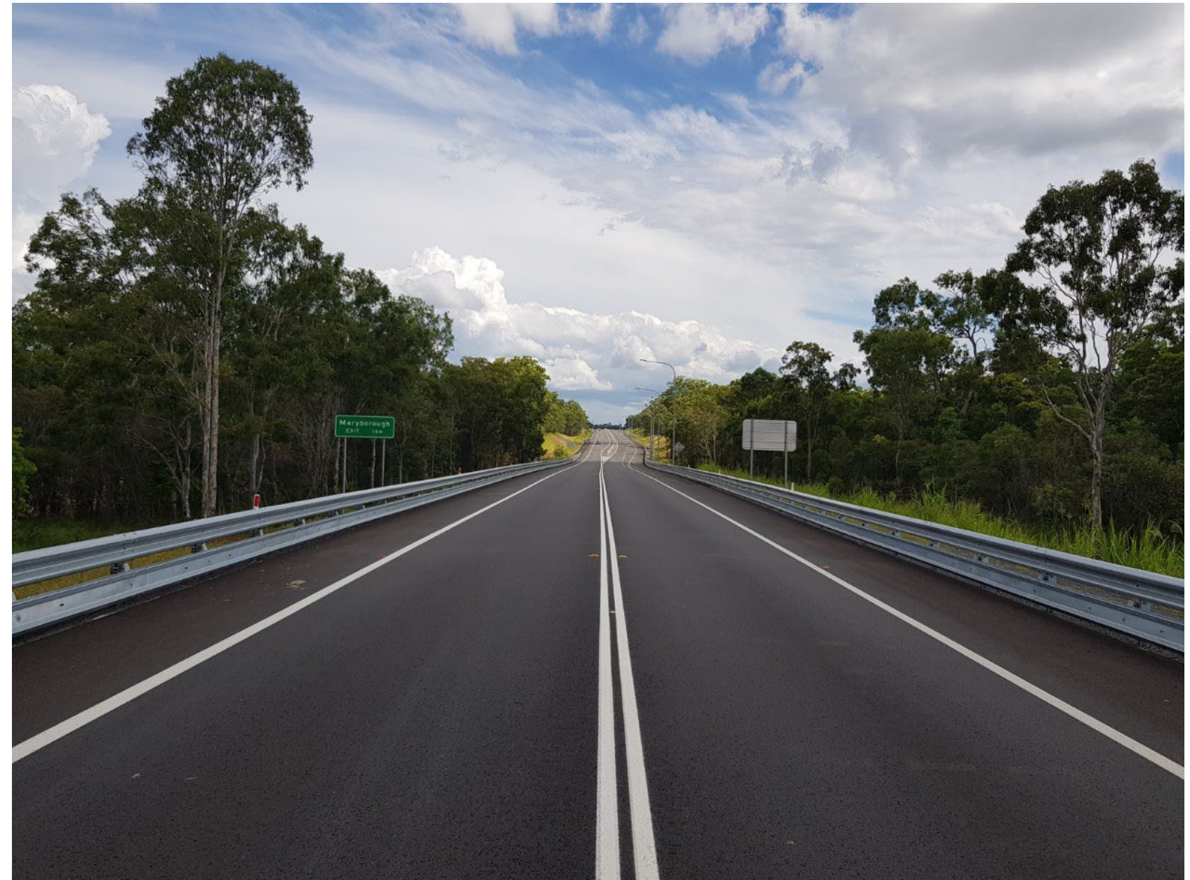
A section of Bruce Highway near Maryborough.
