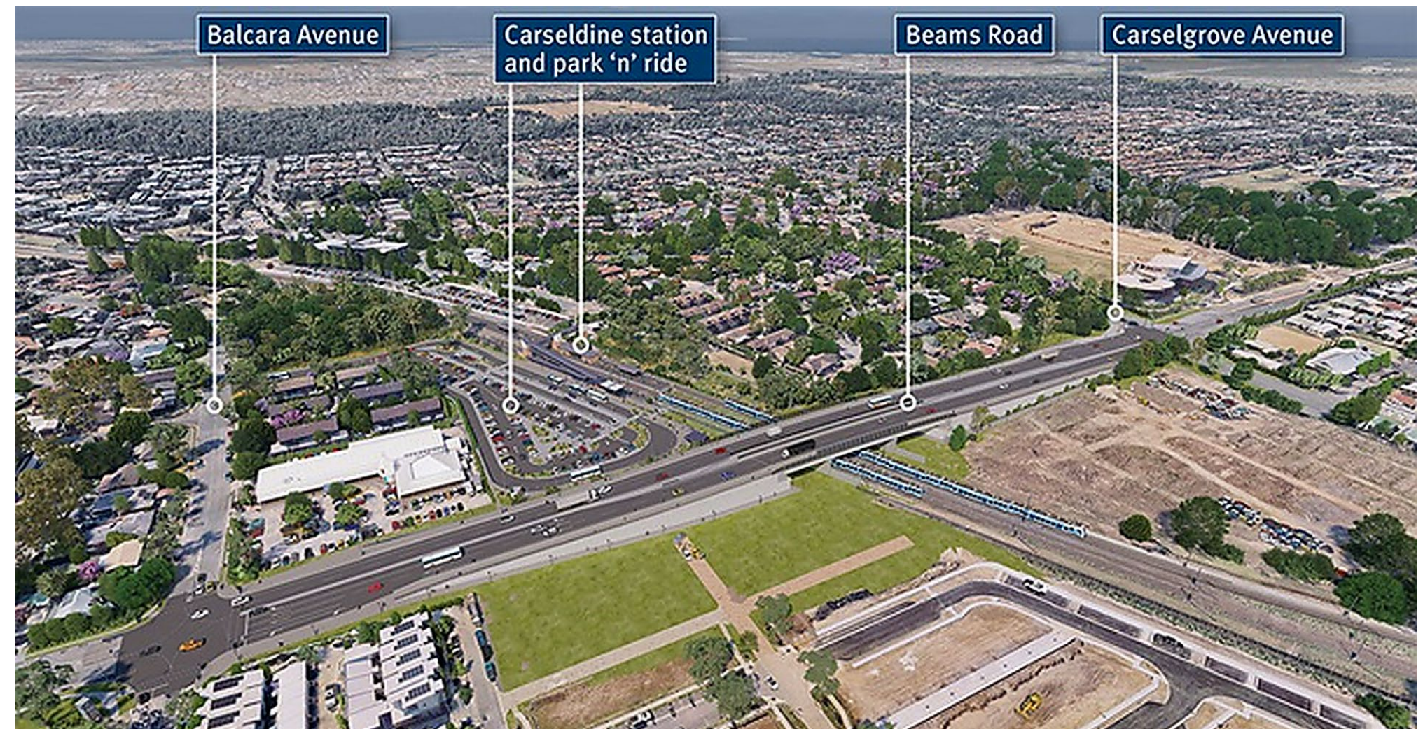
Beams Road rail level crossing upgrade - aerial view looking towards Bracken Ridge
