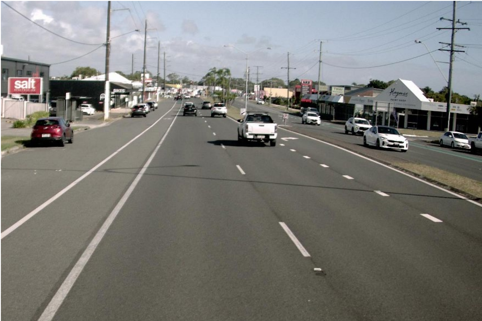
Nicklin Way, Coora Crescent intersection (Currimundi)
