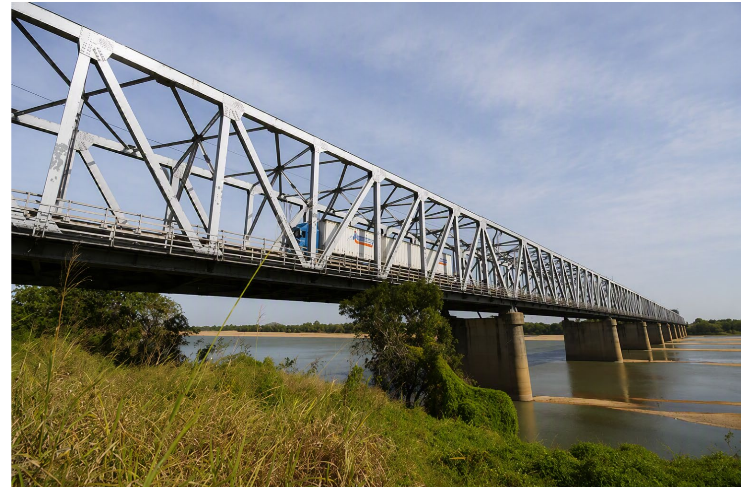
Burdekin River Bridge view from the south-east riverbank
