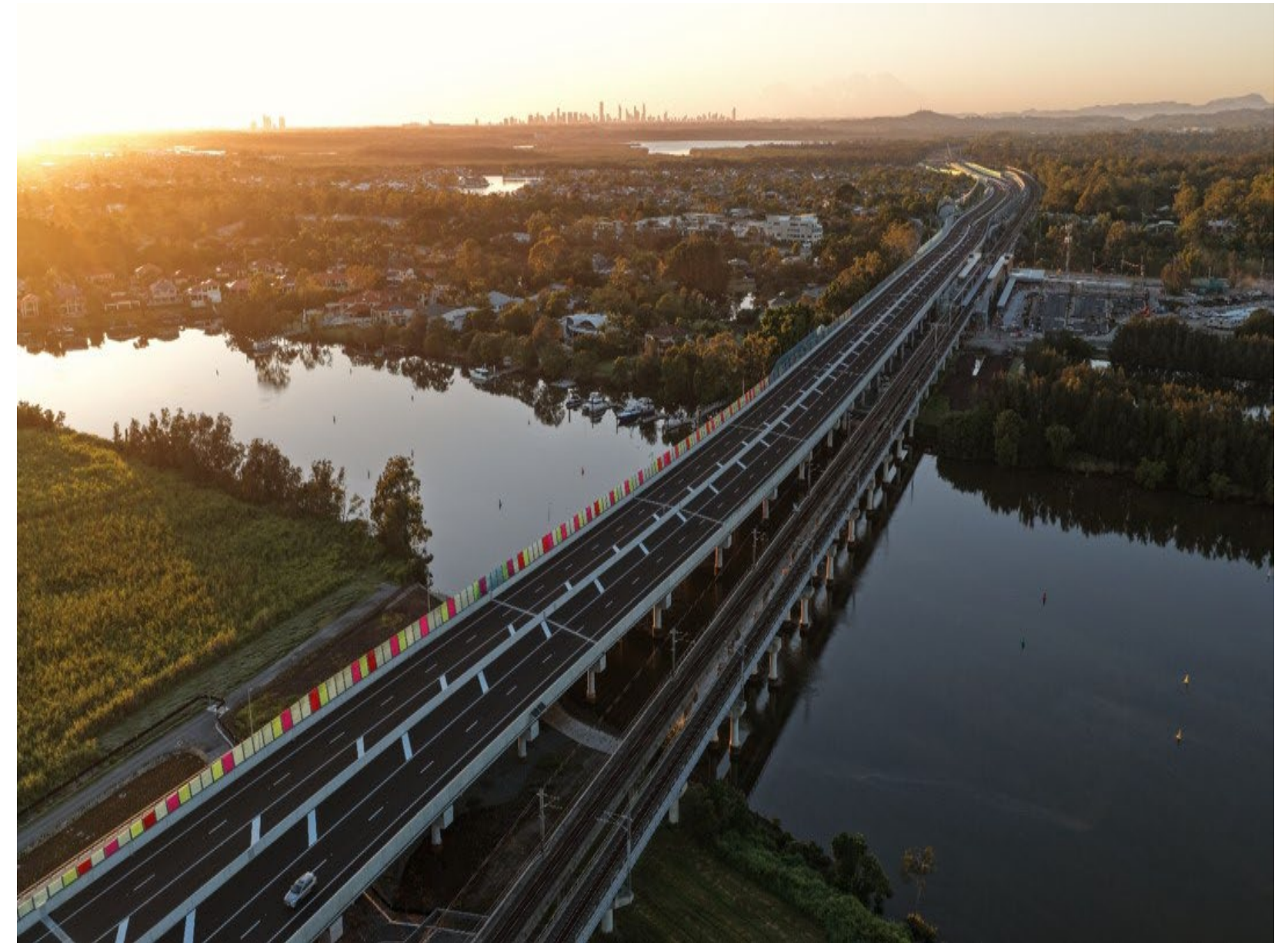
Sunrise over the new Coomera River bridge (Coomera Connector - Stage 1 North), opened to traffic on 2 December 2025
