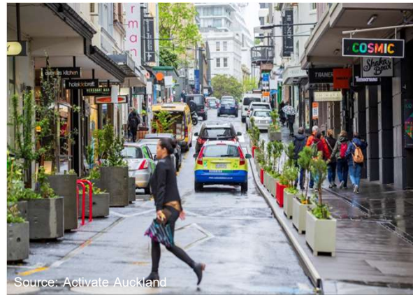
Temporary footpath widening
