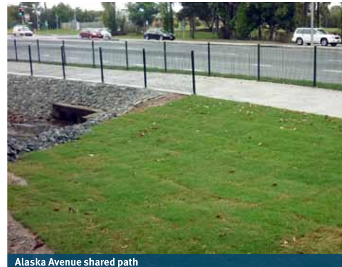
Alaska Avenue shared path
