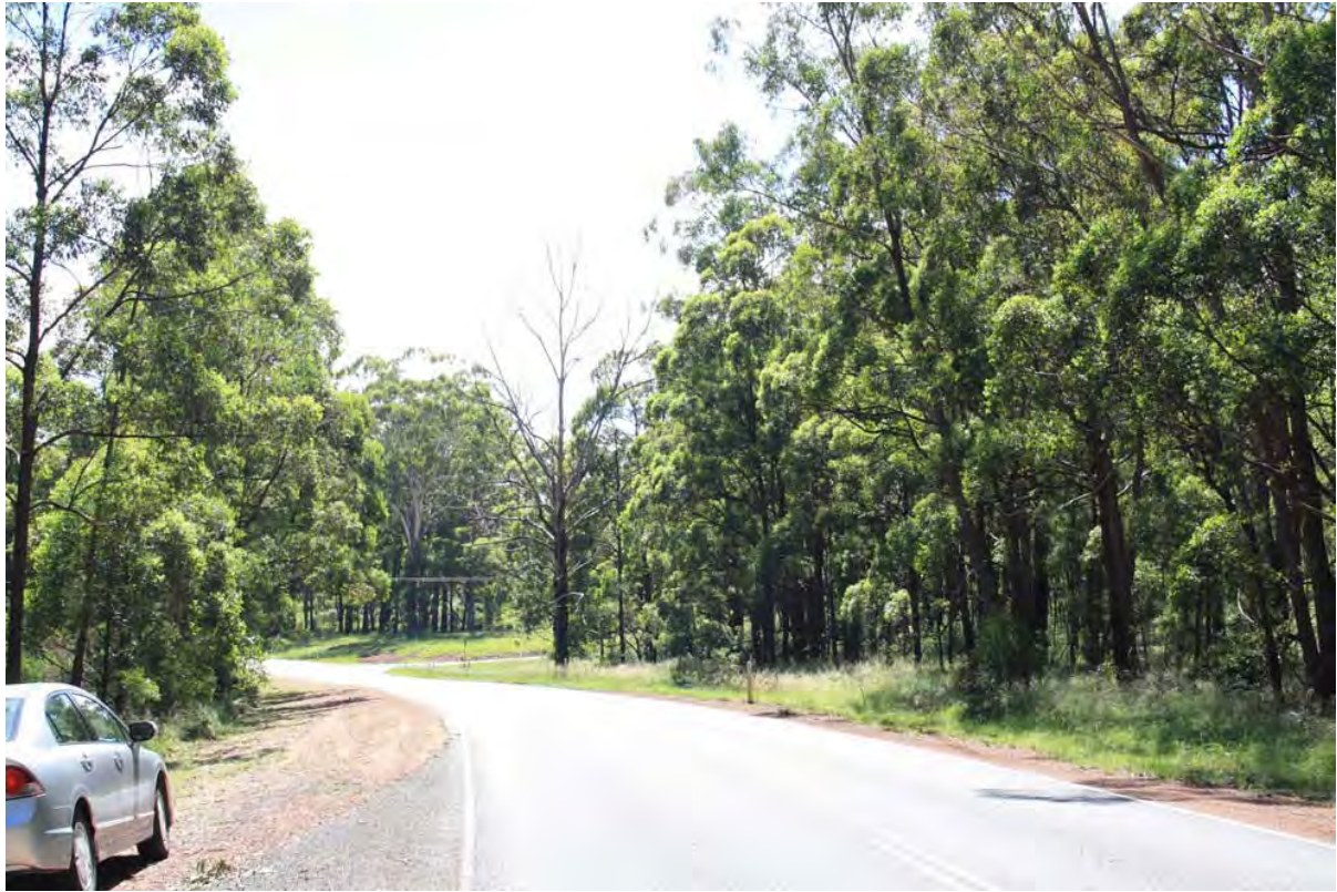
Photo 14 Northbound view, approaching Hampton at Collingwood Road
