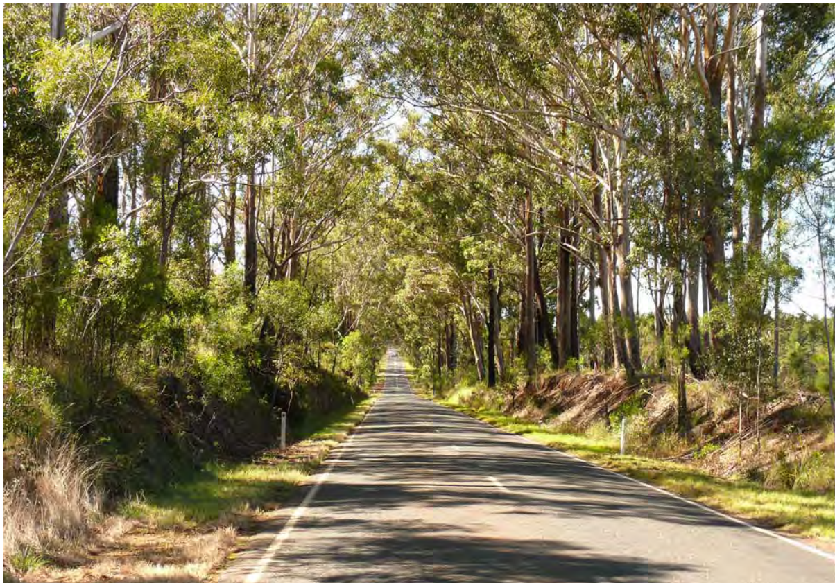
Photo 8 Northbound view, north of Merritts Creek Road
