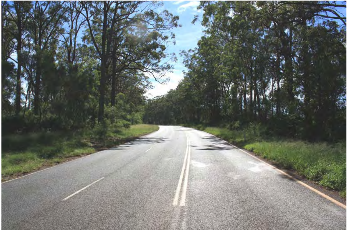
Photo 3 Northbound view, at the start of the northbound passing lane
