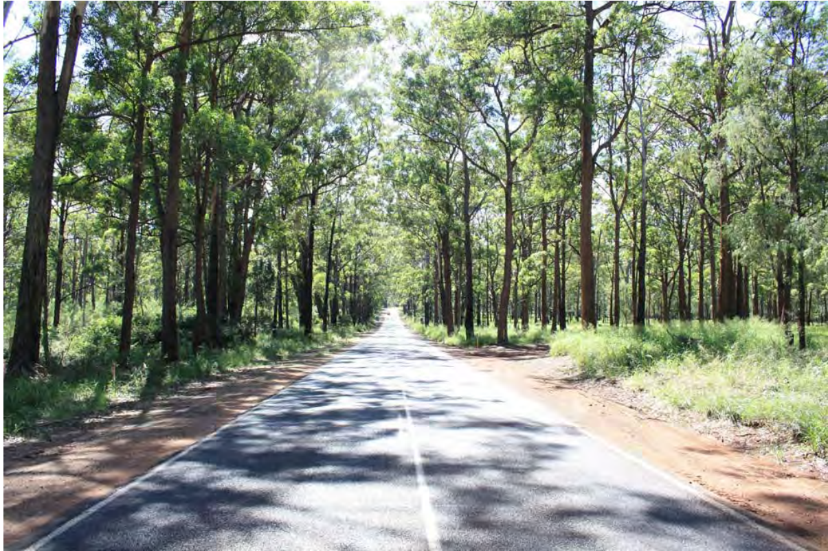
Photo 12 Northbound view, at Keys Road
