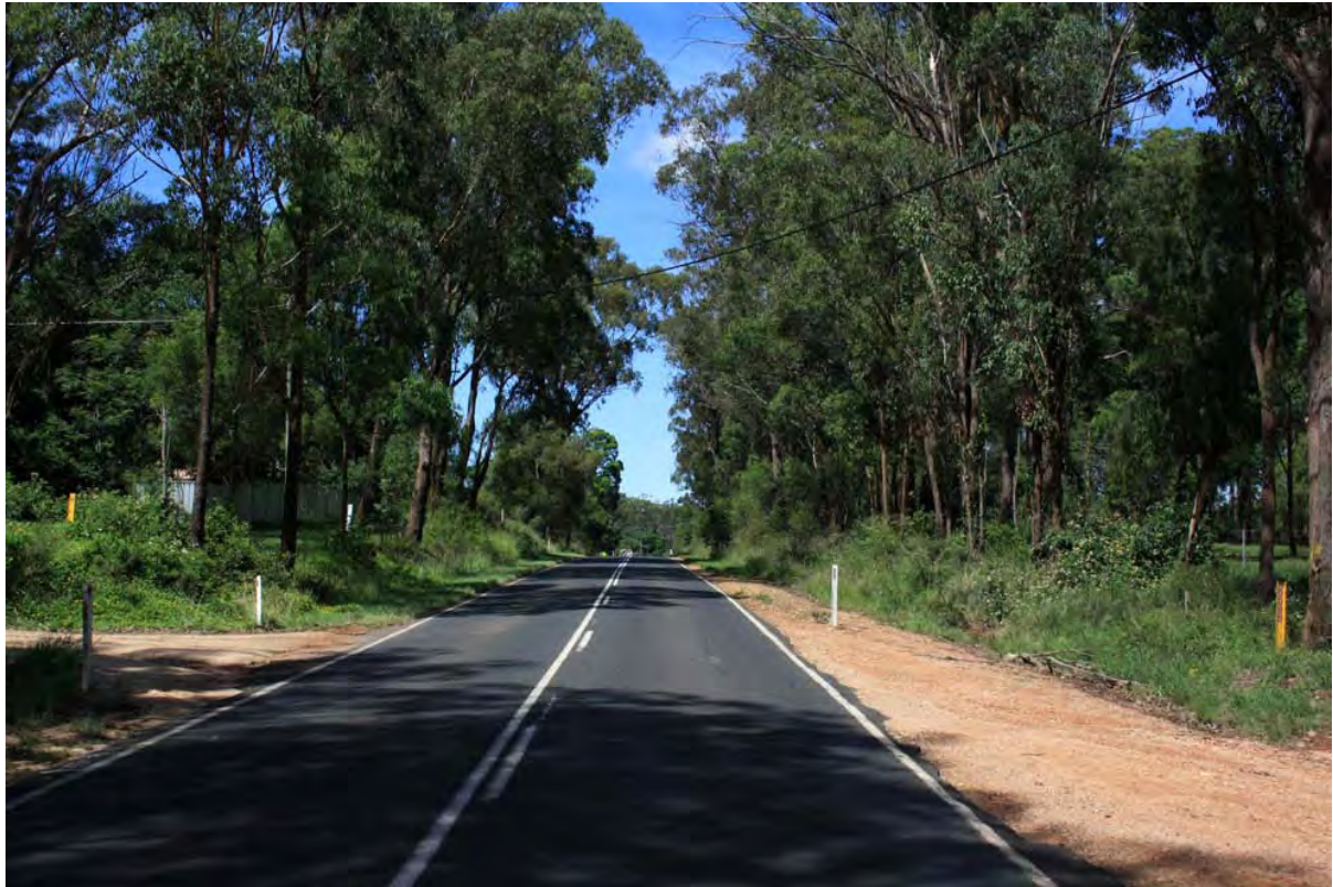
Photo 18 Southbound view, entering Hampton
