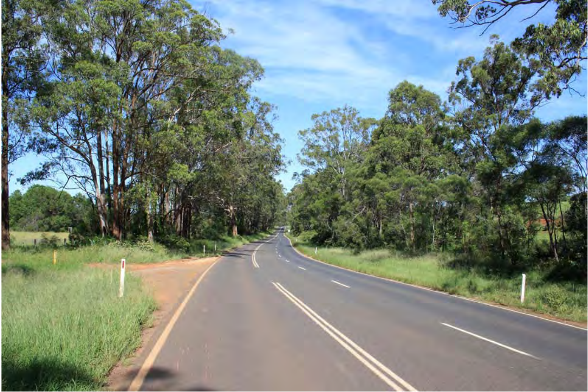
Photo 4 Southbound view, at the end of the northbound passing lane
