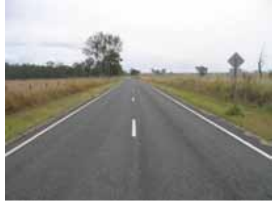
Figure 24 Proposed crossing of Mt Flinders Road - looking west (Ch 25155)
