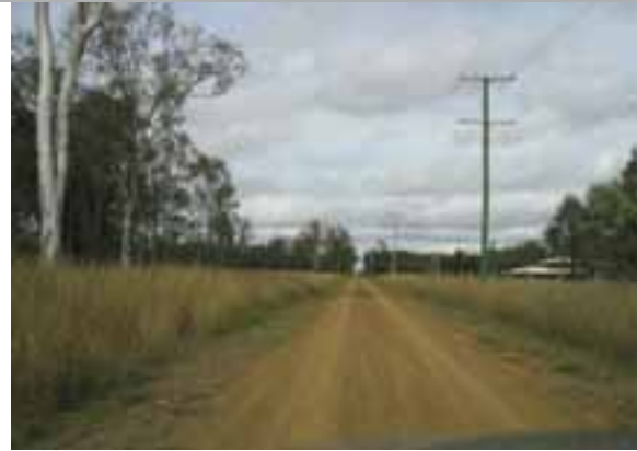
Figure 18 Photo taken in the vicinity of proposed intersection (closure) with M Hines Road (Ch 10455)
