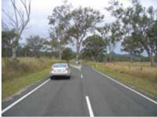
Figure 23 Proposed crossing of Mt Flinders Road - looking east (Ch 25155)
