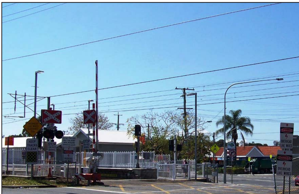
Figure 11: St Vincents Road level crossing
