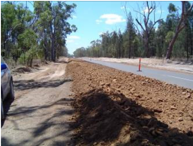
Photo: Widening of the Carnarvon Highway
