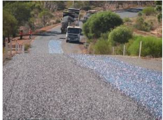
Photo: Contractors resealing roads in south west Queensland
