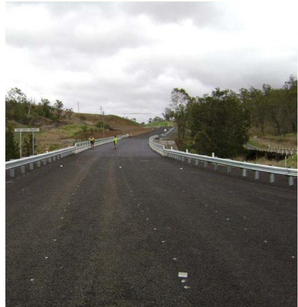
The new Fat Hen Creek bridge.
