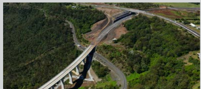
TSRC viaduct to New England Highway
