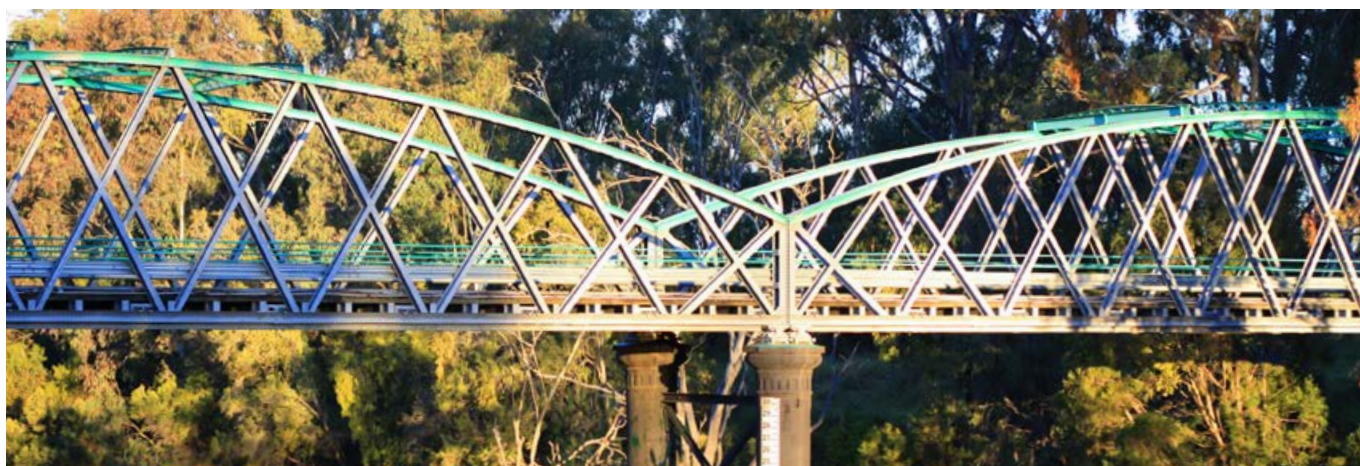
MacIntyre Bridge, Goondiwindi
