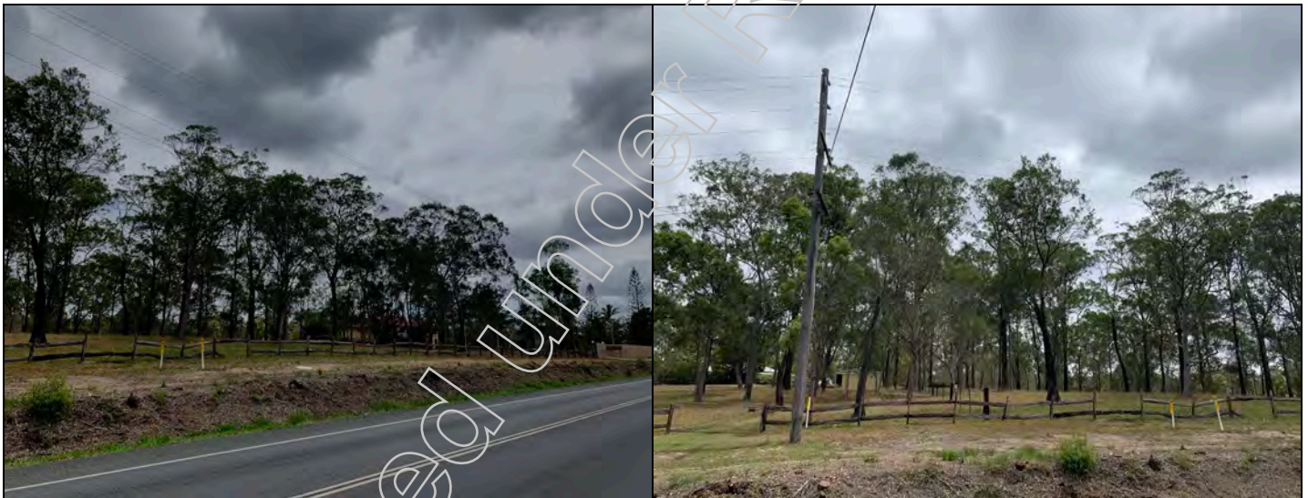
Mapped RE 12.11.27 on western side of Mount Cotton Road, absent understorey, road reserve has been cleared
