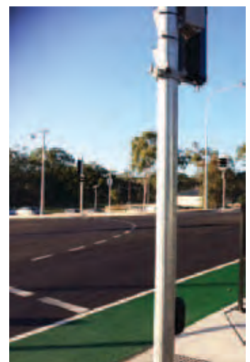
After - Pedestrian muster area including fence and signals adjacent to intersection
