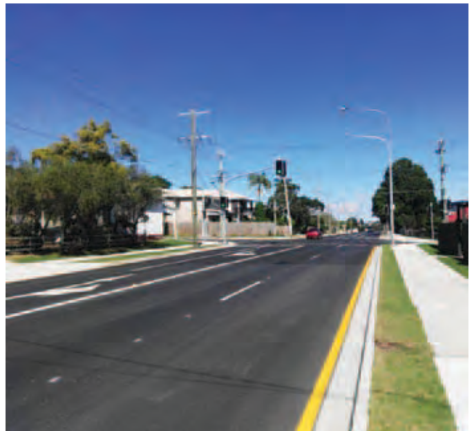
After intersection upgrade
