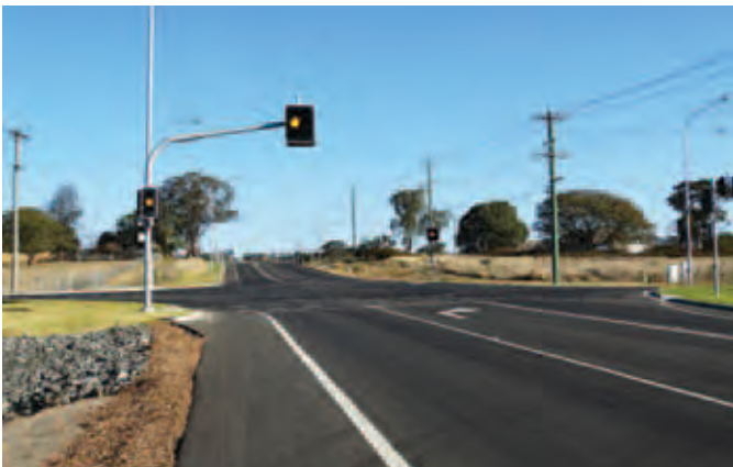
Boundary Street Stage 3 – post construction
