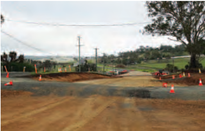
Boundary Street Stage 3 – during construction
