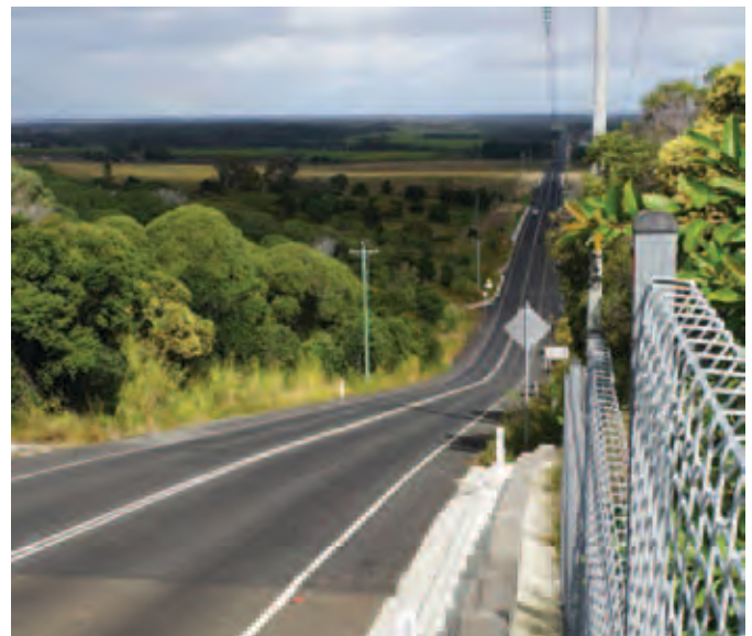
Completed works - View from Stage 3A to 3B
