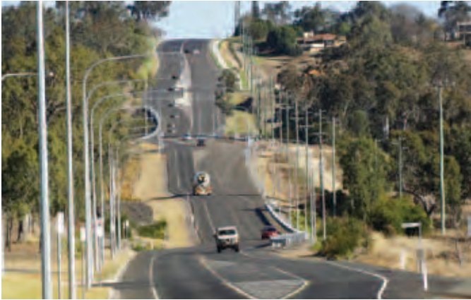
Boundary Street Stage 2 – post construction
