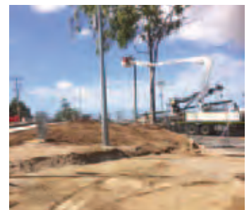
During - Removal of redundant pole by Ergon
