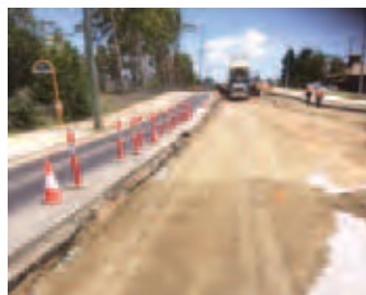
During - Pavement placement including unsuitable remedial works
