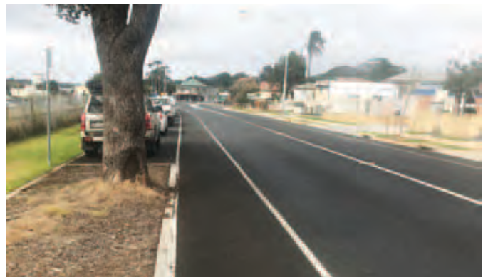
Mort Street – post construction
