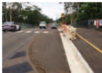
Before - Crest of hill/Centre of new intersection – looking south Preconstruction
