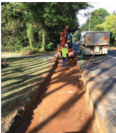
Redlynch Road during/after
