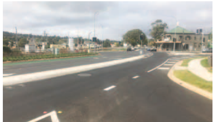
Fiveways intersection – post construction
