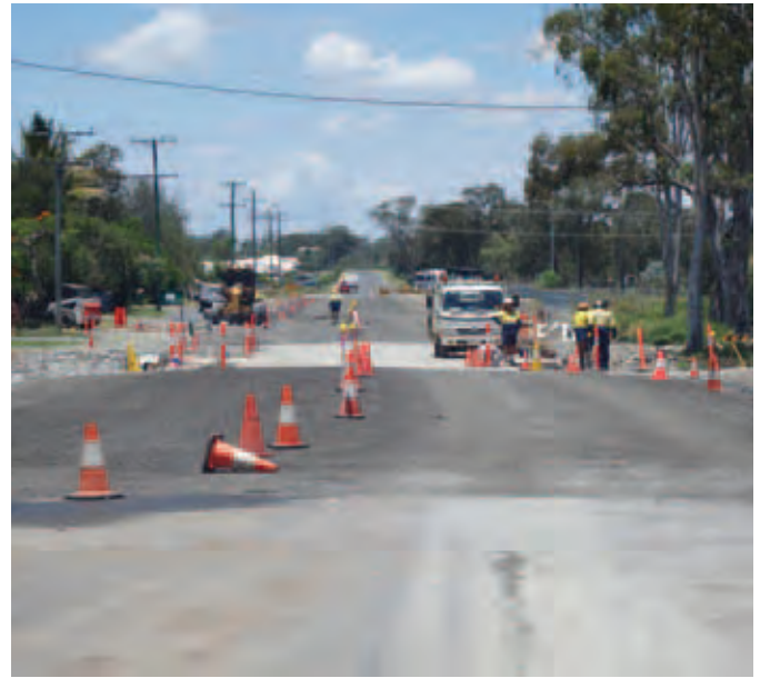
During (Looking to the culvert and further to Middle Road)
