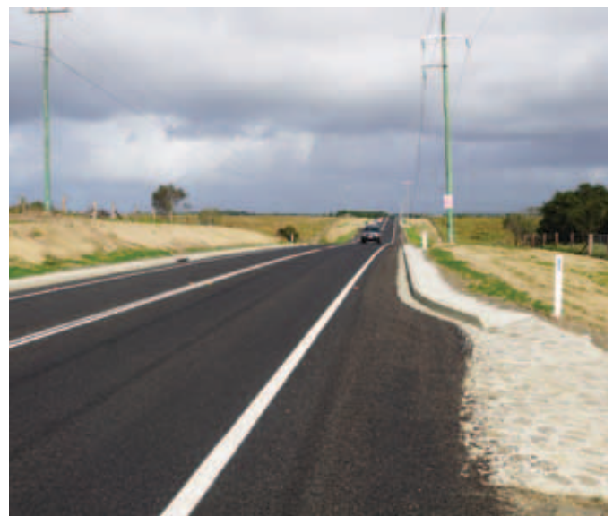
Completed works Stage 3B
