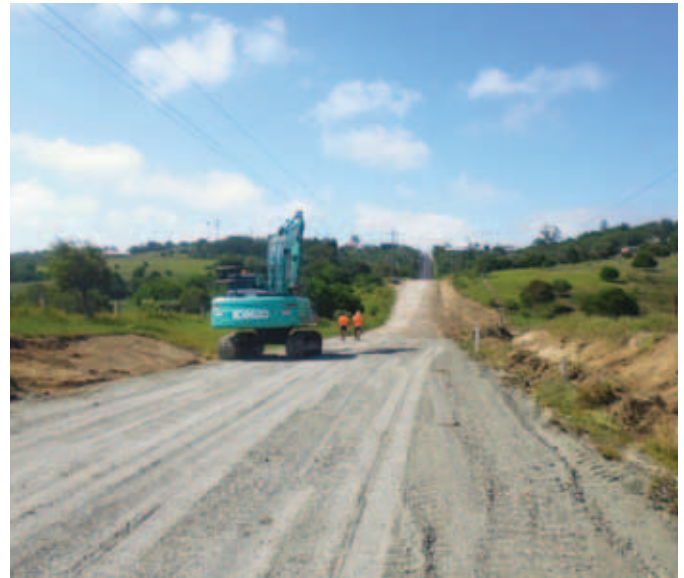
Stage 3B works in progress
