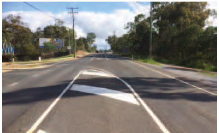
Before - South end of project adjacent Sundowner Drive intersection – Preconstruction
