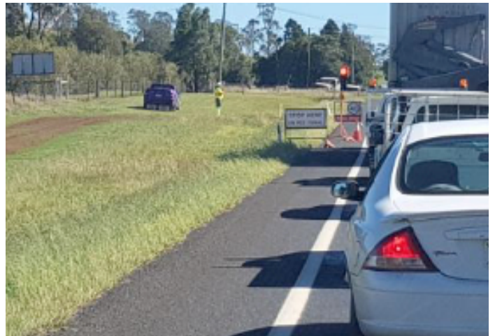
Example of TC operating PTCD from an appropriate location
