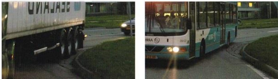
Outside aprons. Note cobbles not preferred due to maintenance, durability and constructability.
