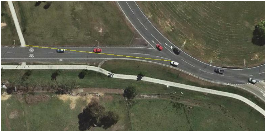
Yellow line indicates path user sight line, third approaching car potential not visible to path user. Robina Parkway at Gooding Dr, QLD
