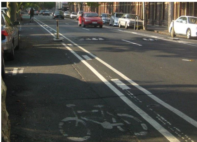
Speed cushion and splitter kerb used in combination. Yarra VIC
