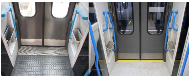
Figure 2.5 - A before (left) and after (right) example of refurbished doors with colour-contrasting floor and accessible handrails. Note that the access path in the before image contrasted better with the walls.
