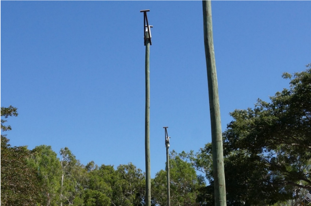
Figure 6B-1 – Purpose-built glider poles with launching arms to provide glider species passage across the road
