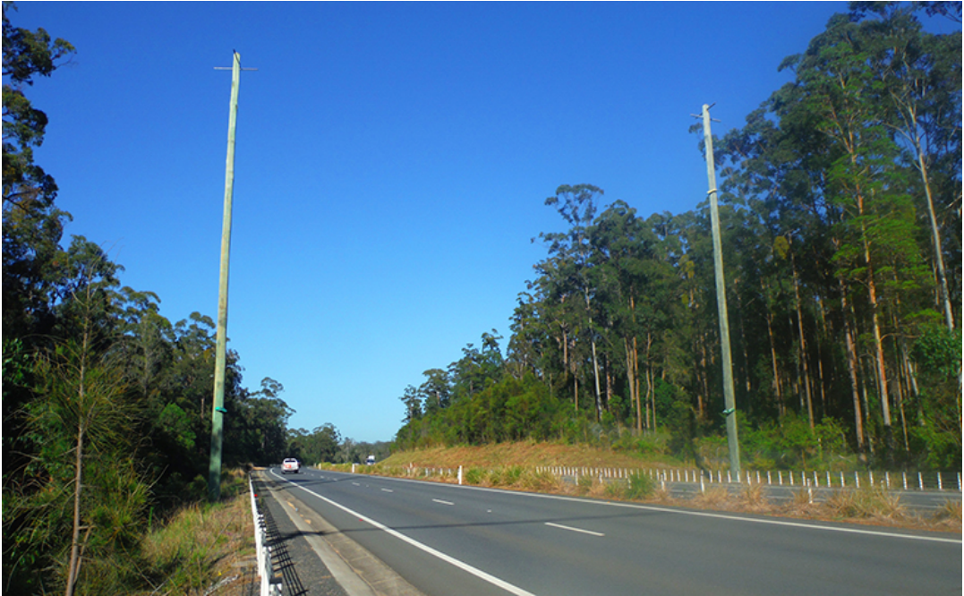
Figure 6B-2 – Glider poles installation along road with safety barriers
